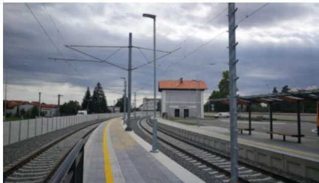
Transfer terminal in Židlochovice
